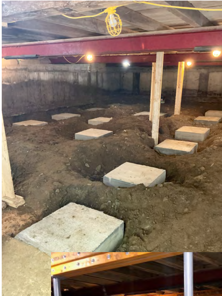
Cultural Center work completed by Larochelle Construction
